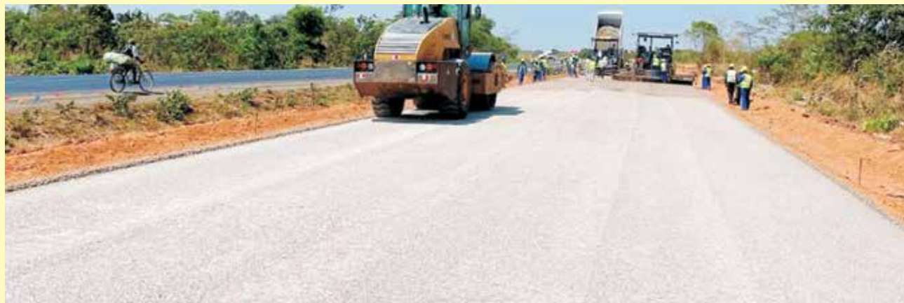
Construction of the Lusaka-Ndola Dual Carriageway
