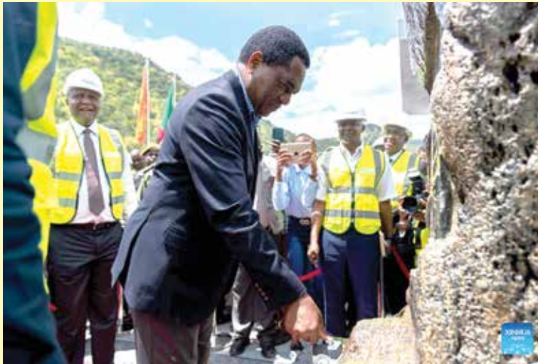
President Hichilema (front) pushes the start button to commission the fifth generator at the Kafue Gorge Lower Hydropower Station
