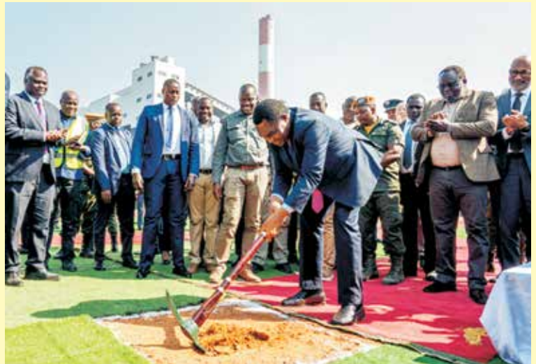
President Hichilema commissioning the 300MW Phase II of the Maamba Power Expansion Project
